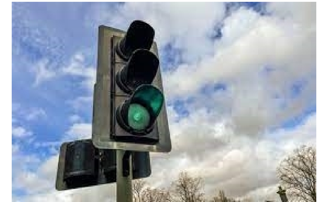
Signal priority for late running bus giving a green wave through signals
