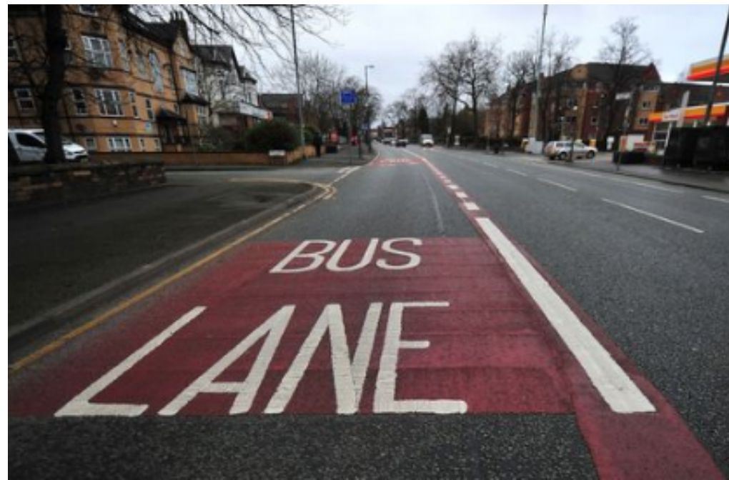
Bus Lanes where there are points of delay for bus caused by traffic congestion and spare road space exists
