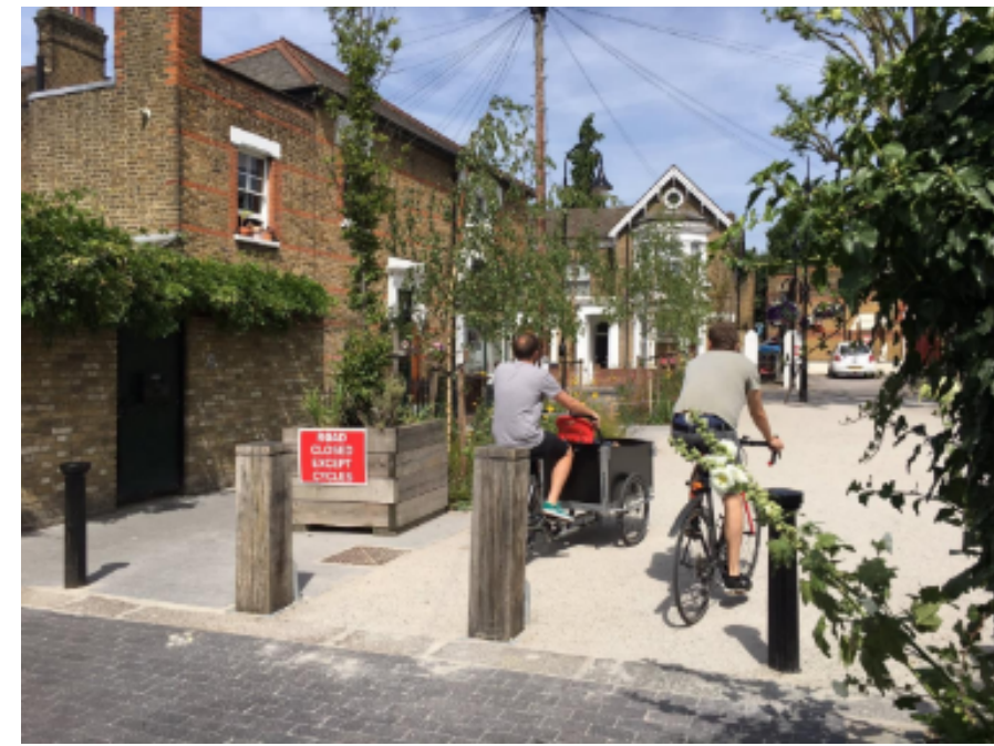
Active neighbourhoods that support local trips by foot and by bike through side road closures
