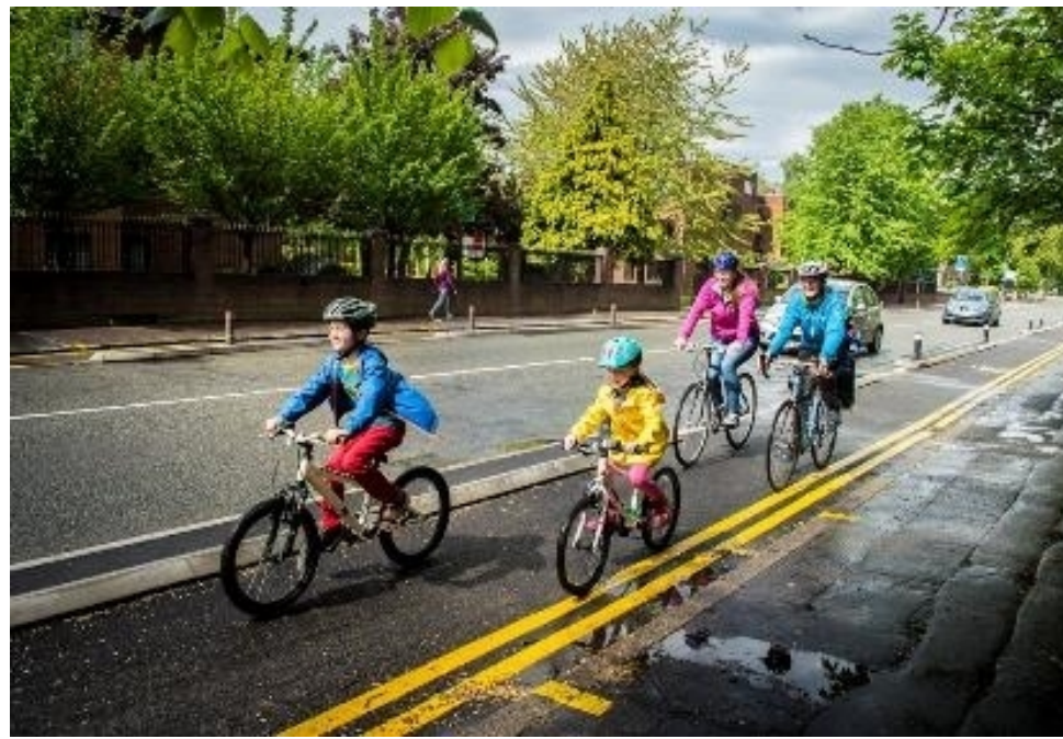
Delivering high quality key road infrastructure that meets local and national standards
